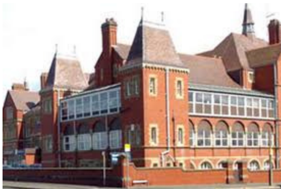
Site of North Denbighshire community hospital development
